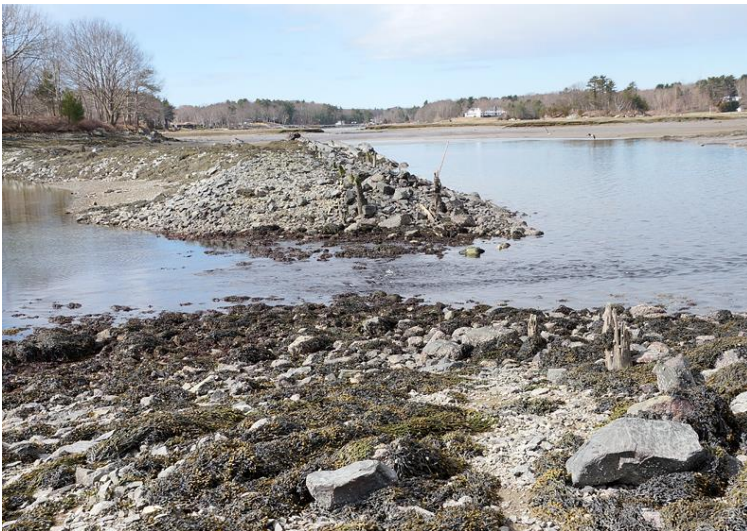
Outflow, left to right, through the low point in the Wentworth mill pond dam, looking toward Sagamore Creek.
