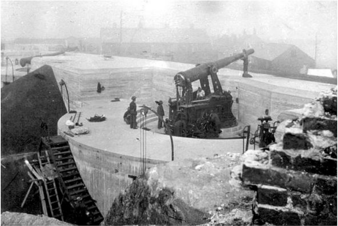
Battery Farnsworth, with the foundation of Walbach Tower in the right foreground. The battery has just been completed, except for the iron railings along the stairs and parapet. The two guns are 8-inch breech-loading rifles, mounted on disappearing-type carriages. The west wall and gate of Fort Constitution can just be made out in the left background through the fog. (from Bolling Smith Collection, via American Forts Network web site)
